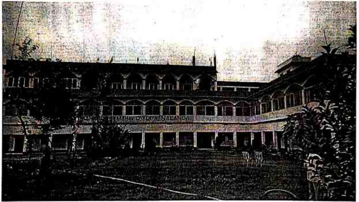
Front view of the Building
